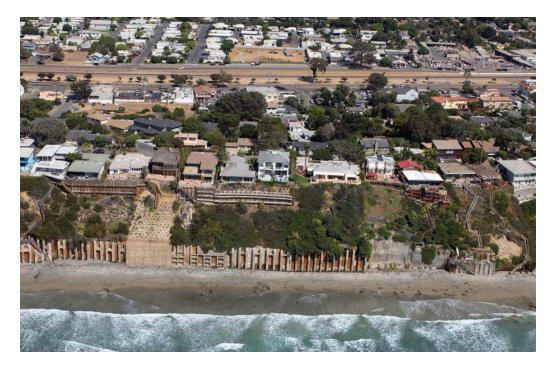
**Figure 9.8 Coastal armoring in Southern California.** One-third of the shoreline of Southern California (including Ventura, Los Angeles, Orange and San Diego Counties) has now been armored. The photo shows the shoreline in 2010 in Encinitas, in northern San Diego County. Photo courtesy of Kenneth and Gabrielle Adelman of the California Coastal Records Project (http://www.californiacoastline.org/).
